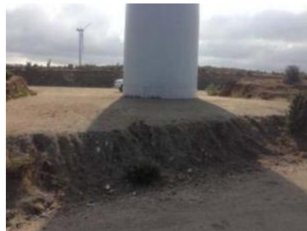
Figure 7.8. WTG 3 Foundation showing backfill
