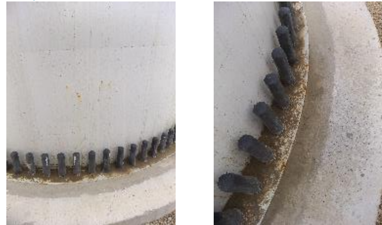
Figure 7.17. Inspections for tower connection to foundation
