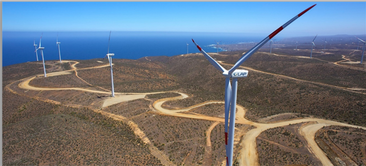
Aerial view of Totoral wind farm.
