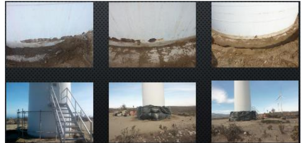
Figure 7.5. Example coating repairs (2019)
