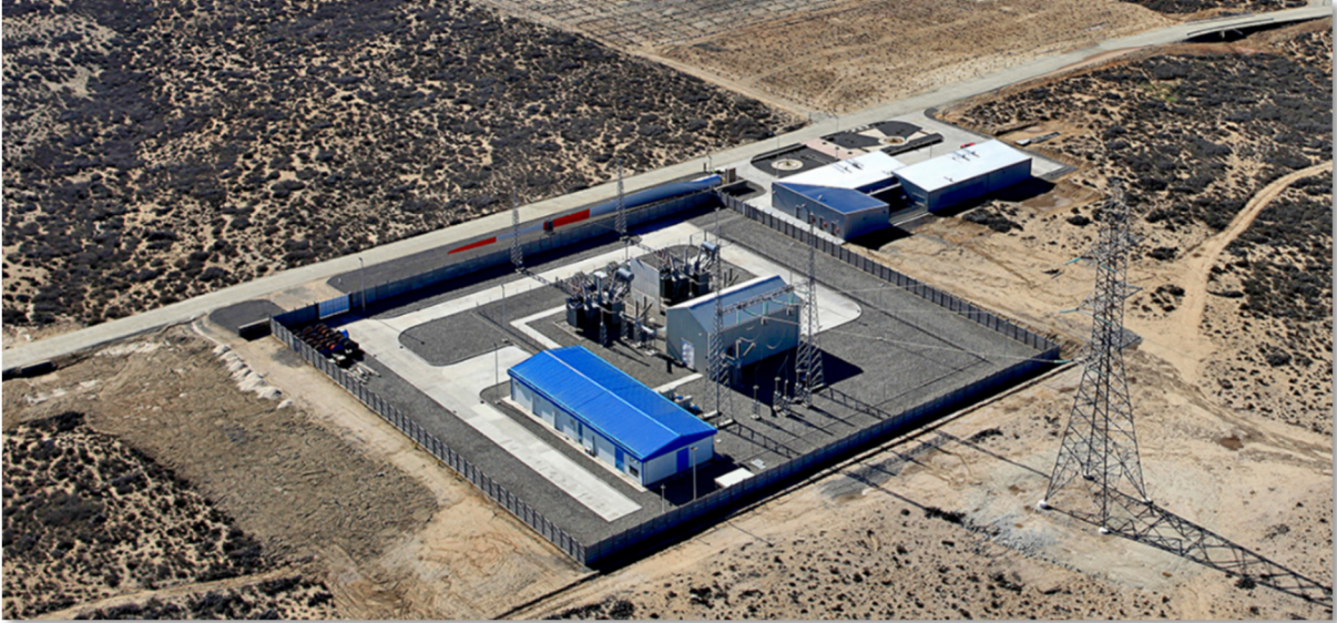
San Juan Substation & control office.
